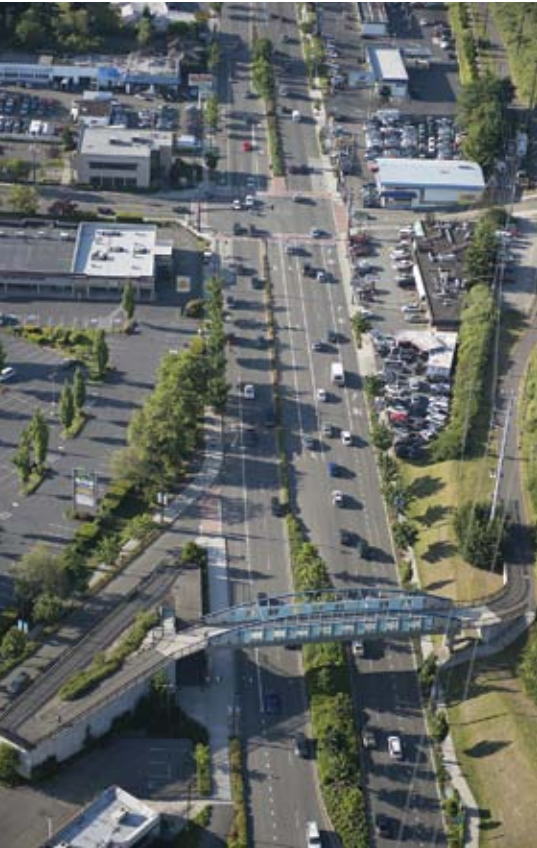
Improvements along the Aurora Corridor have included a new pedestrian bridge, landscaped medians, and upgrades to utility infrastructure. (HDR ENGINEERING INC.)
